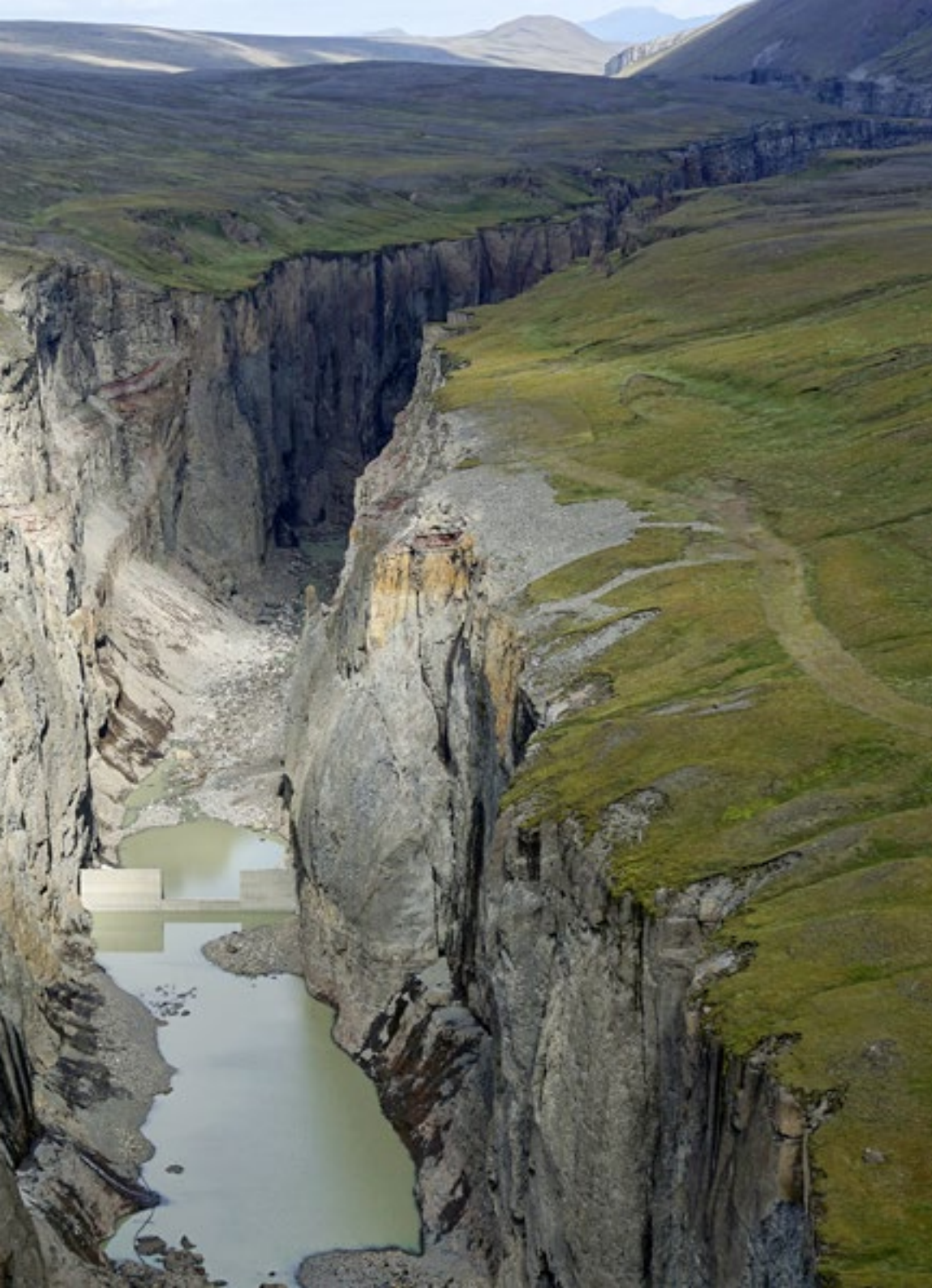
Kárahnjúkar hydroelectric dam in the eastern highlands of Iceland.
